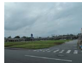
After the dismantling of the buildings
