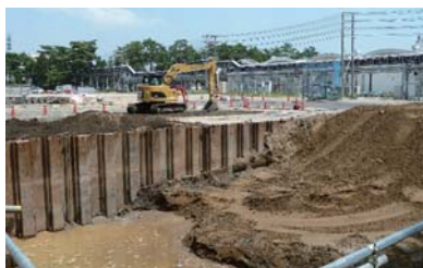
A scene from the excavation work on the contaminated soil
