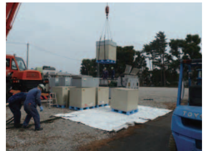
Scene of PCB waste being removed
