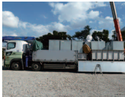
Scene of PCB waste being removed
