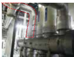
Cool water header newly connected bypass
