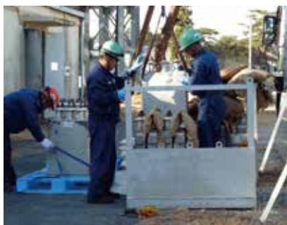
Loading to dedicated truck (1)
