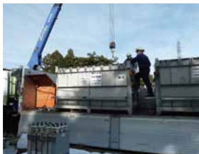
Loading to dedicated truck (2)
