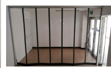
at entrances to changing rooms Installation of thermal curtains
