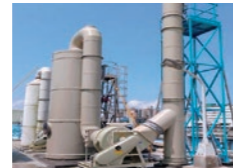
Installation of an additional VOC wet scrubber *VOC: Volatile Organic Compounds
