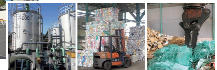
Storage tanks for flammable waste oil
