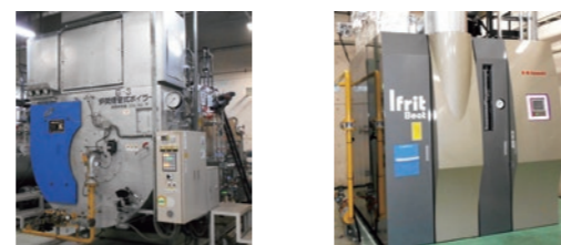
Smoke-tube Boiler → Once-through Boiler
