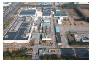
Full View of Solar Panels
